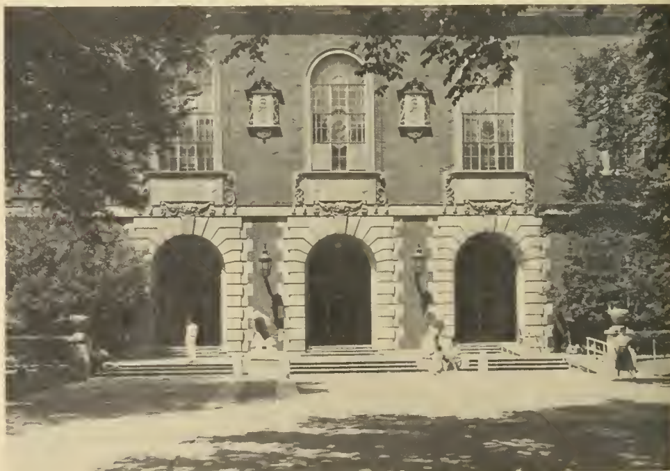
The east entrance of the University of Illinois Library.
